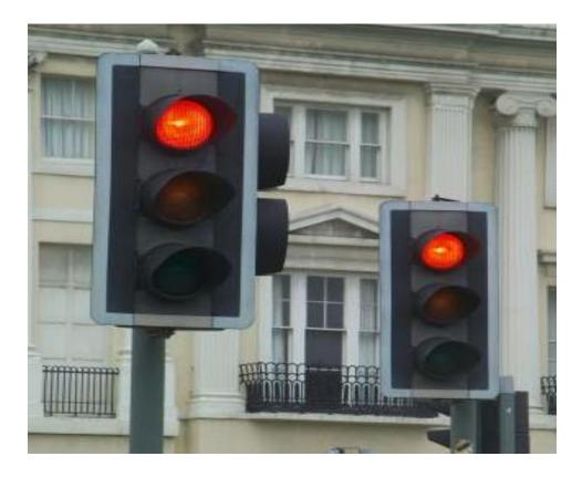
The amount of time provided for the all-red interval is very much a matter of local preference and the peculiarities of the individual intersection. However, except at very wide or unusual intersections, the all-red interval typically ranges between 0 (no red interval) and 2 seconds.
